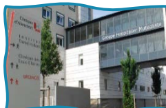
Private not-for-profit hospital, Grenoble
