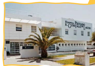
Lagos private hospital, Portugal
