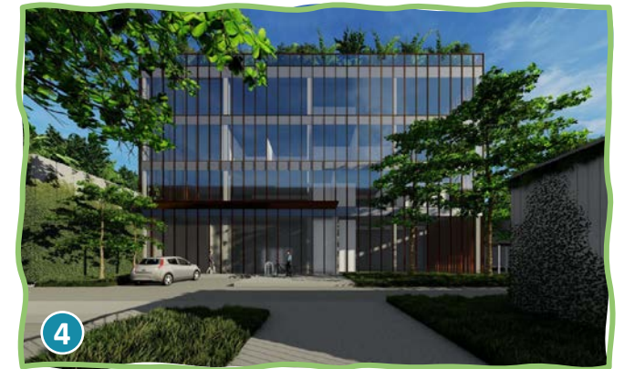
Equinix datacenter project
