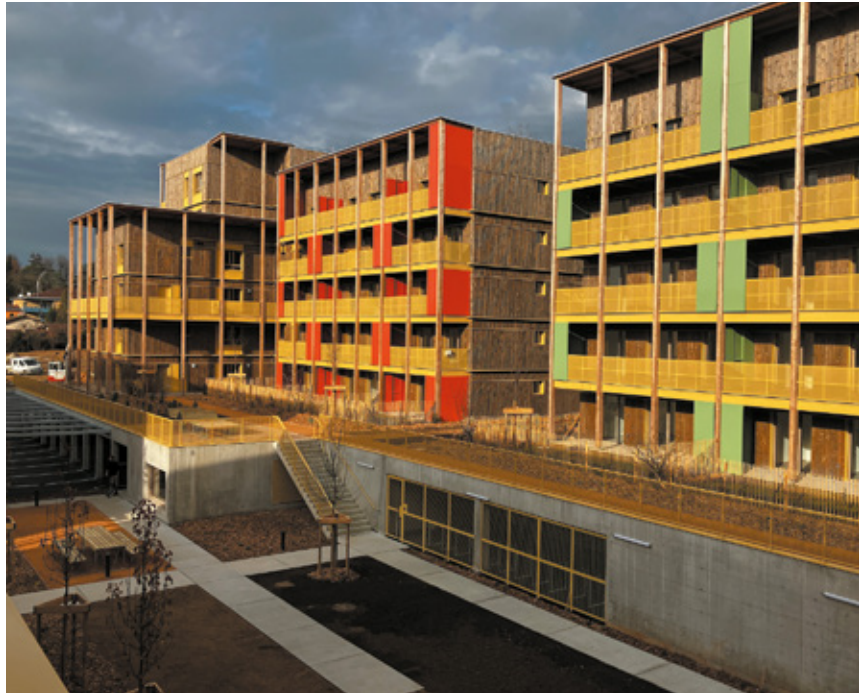
Origine, Trévoux (Rhône). A complex with 84 residential units and a guest house designed to resist higher temperatures, particularly through the use of wood which helps to cool the apartments in summer and conserve heat in winter.
