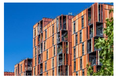
The Wood'Art building in Toulouse (Haute-Garonne), with 76% of its structure made from wood
