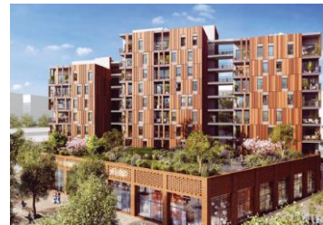
The 76% timber-based Wood'Art-La Canopée complex in Toulouse (Haute-Garonne)
