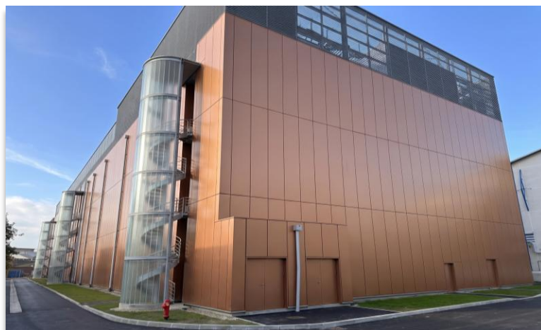
EQUINIX DATA CENTER (Portes de Paris business park, Seine-Saint-Denis)
