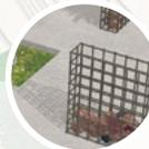
Materials reuse, i.e. the reuse of materials during construction and the second life of materials after construction, has enabled the Athletes Village's carbon footprint to be drastically reduced. Following the Games, materials used for interior elements, such as temporary partitions, carpeting and paint, will be reused. Outdoor reuse initiatives include the use of ceramic scrap to create gabion walls and the recovery of wood from northern Europe (Netherlands) to make outdoor furniture.
