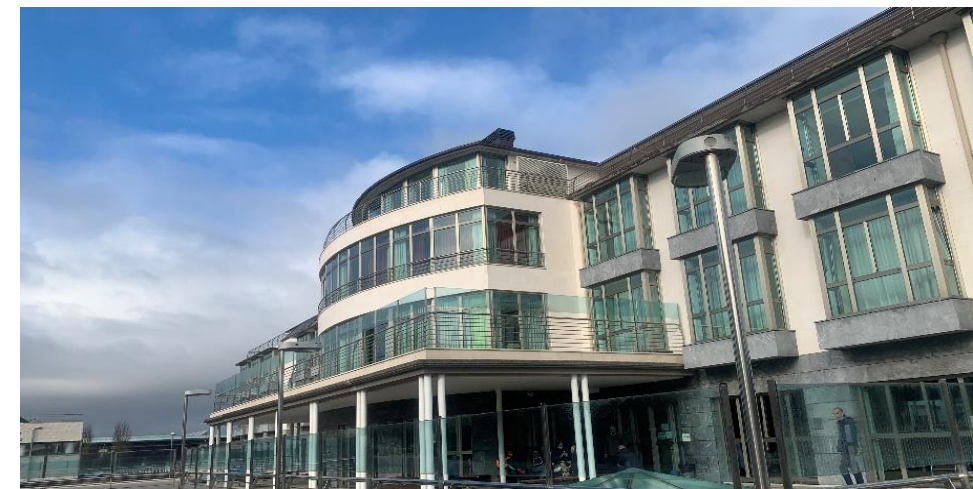
LONG-TERM CARE FACILITY, Spain
