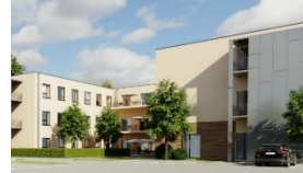
Durlangen nursing home, Germany
