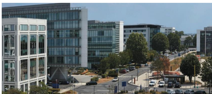
ORLY-RUNGIS BUSINESS PARK, Val-de-Marne
