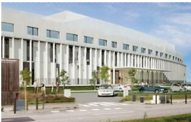
FRC facility (Toulouse, Haute-Garonne)
