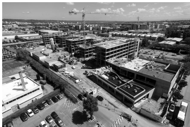
Silky Way Project – Construction site, end of 2014
