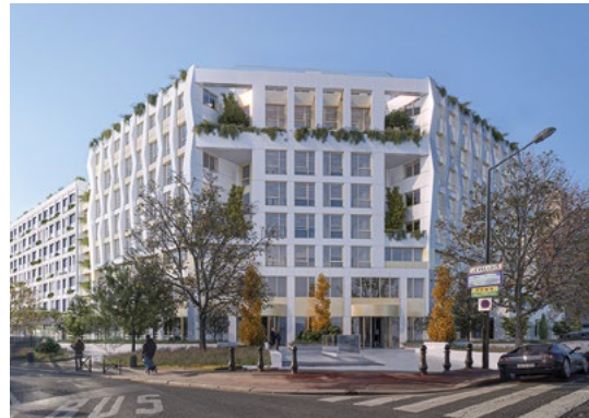
City Park in Levallois-Perret (Hauts-de-Seine), developed by AfterWork by Icade, JP Morgan Asset Management and Semarelp. Architecture firm: DGM & Associés
