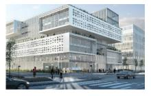
The building is located on the Avenue de France, directly opposite the Simone de Beauvoir footbridge and the National Library of France. Developed by Icade and designed by Marc Mimram, this bridge-shaped, fully steel-framed building spans the railway tracks of the Austerlitz station over 58 metres—a true engineering feat.
