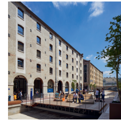
LE CAMBRAIS - 025 BUILDING
